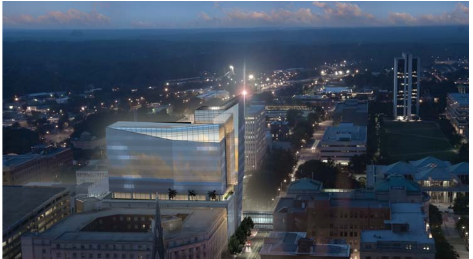
Photo Composite View, (North Carolina) State Employee's Credit Union, Raleigh, NC, O'Brien/Atkins Architects, Research Triangle Park, NC
