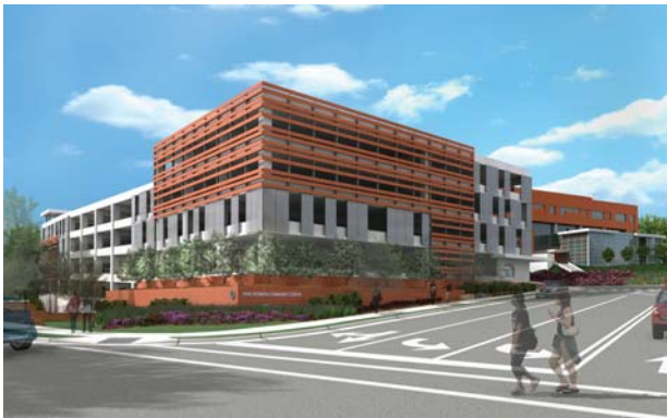
Wake Technical Community College Parking Structure, Raleigh, NC, BBH-Design, Research Triangle Park, NC
